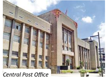
Central Post Office
